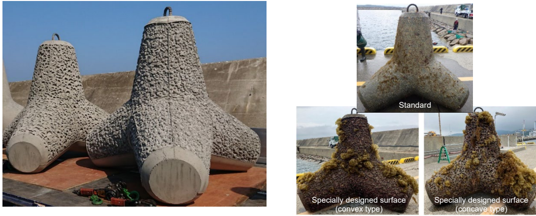
Figure XX J Blue Concrete blocks with specially designed surface shapes
