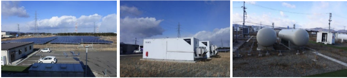
Figure 14. Equipment used at the SIGC: (from left to right) solar power generation facilities, battery system, and hydrogen tanks
