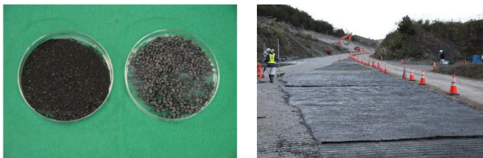
Figure 27. Powder and granular biochar (left) and application to an actual construction site (right)
