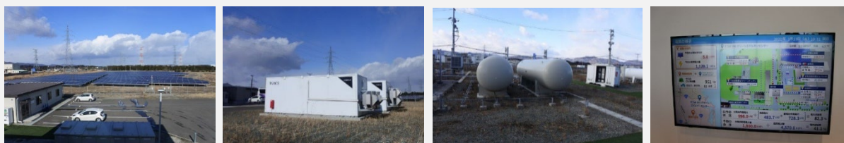
Figure 15. Equipment used at SIGC: (from left to right) 1.6 MW solar power generation facilities, battery system, hydrogen tanks, energy management system screen
